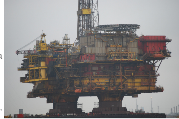
The 24,200-tonne topside of the Shell's Brent Delta oil and gas platform, located in the North-East coast of Shetland (UK) in the North Sea, was decommissioned and removed in April 2017. Photo by Kevin Harris on Unsplash .
